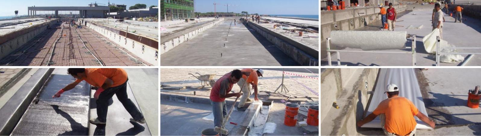
*“ The pool surfaces were laminated with CSM, and then METYX Composites peel plies were used to prepare the surfaces for the secondary operation, which was an epoxy base coat followed by a polyurethane coating finish. We were able to supply a large quantity of peel plies with very short lead time, enabling our customers to complete the project on-time. Companies with challenging projects can always depend on us to be a reliable partner. ”*
